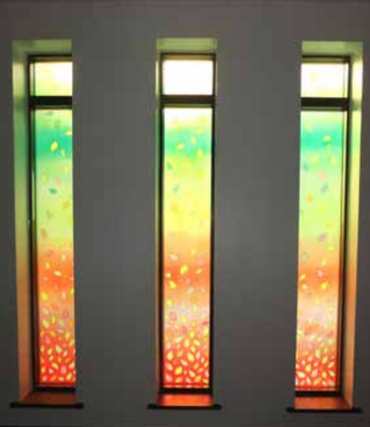
Glass panels for quiet room, Marie Curie West Midlands Hospice, Solihull, West Midlands. Digitally printed optically clear film.
